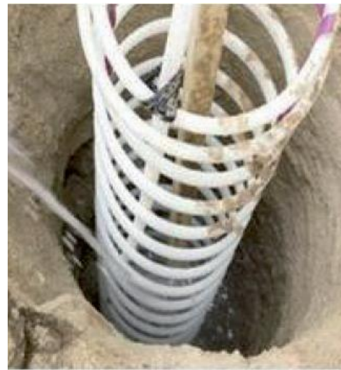
Helicoidal Ground Source Heat Exchangers
