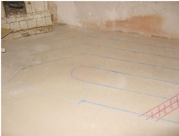
The result of surveying was drawn on the floor surface by chalk.
