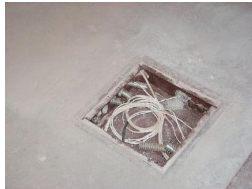
Wells with cables in the concrete floor.
