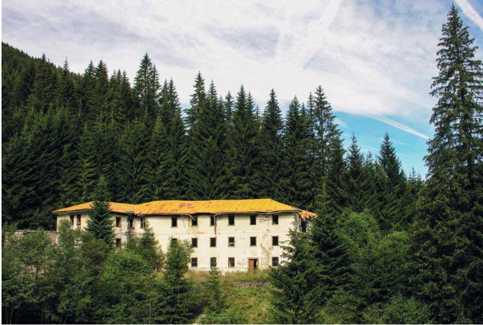
Fig. 4 - On the Lagorai range, “between two mountains, not far from each other formed of red porphyric-quartzitic rock” (in reality, of riolithic or riodiacitic ignimbrite), in the valley of Cavelonte, in the municipality of Panchià (TN), one can see the ruins of the building (built in 1850) of Cavelonte’s spa. Its ferruginous or vitriolic waters, discovered in 1754, were appreciated for their disinfectant and anti-inflammatory action, trophic on the mucous membranes; stimulating on the epithelial cells, muscle-relaxing, stabilizing mood tone. They were analyzed by D. Leonardi in 1831.
